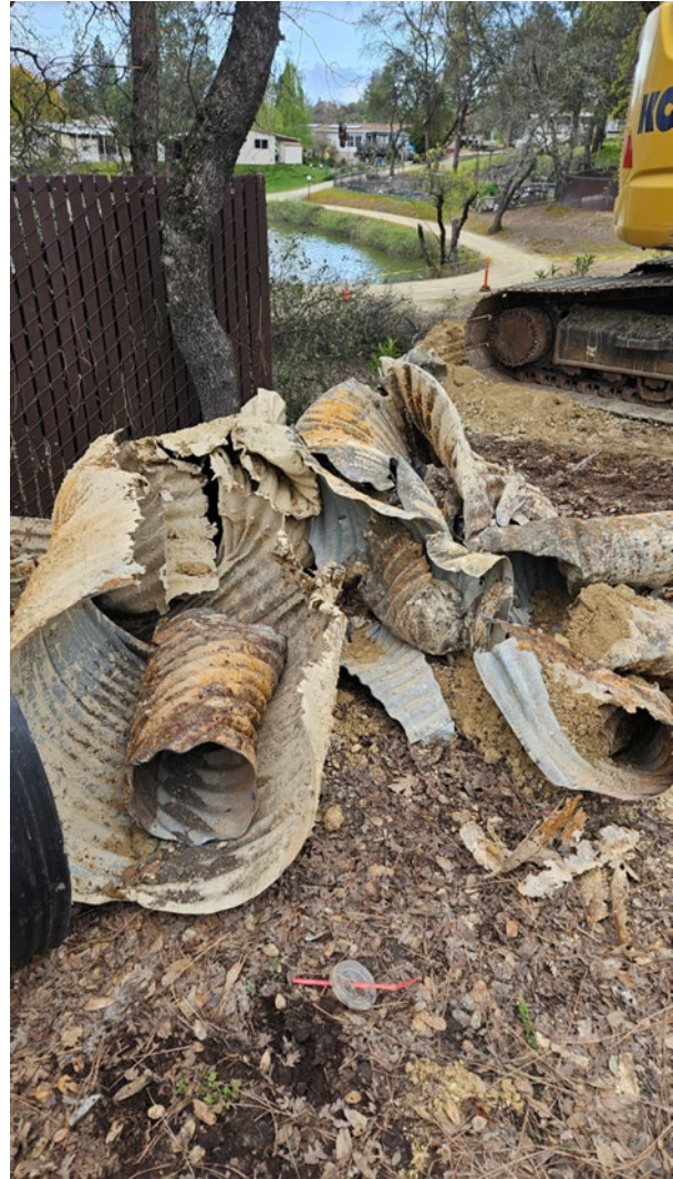
Damaged/destroyed culvert removed from roadway
