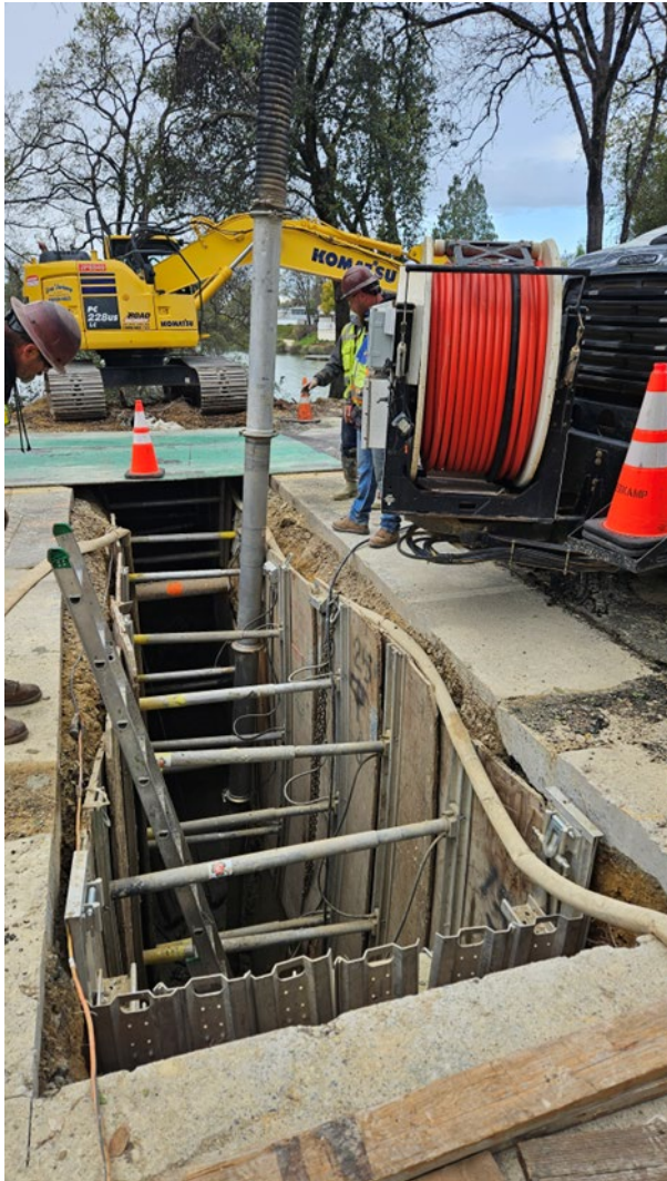
15' deep culvert excavation under Patterson Drive
