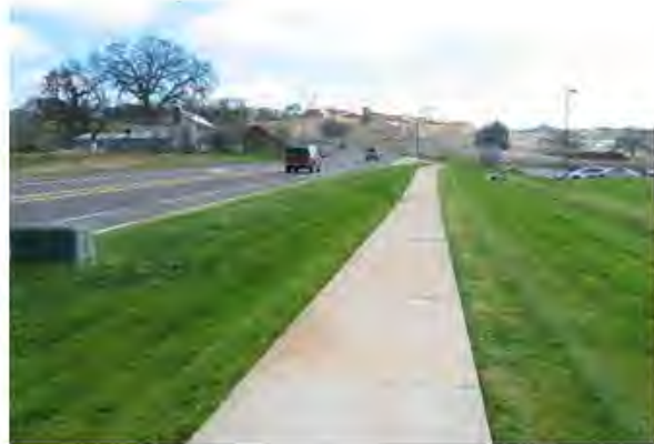
A separated sidewalk along Green Valley Road in front of Pleasant Valley School provides a safe and comfortable walking experience for users.
