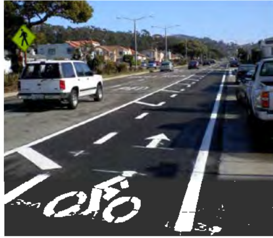
The use of pavement markings delineates space for bicyclists to ride in a comfortable facility.
