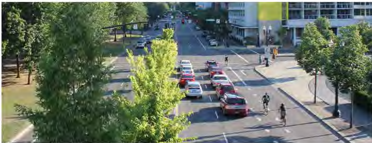
Drivers wishing to enter the right turn lane must transition across the bicycle lane in advance of the turn.
