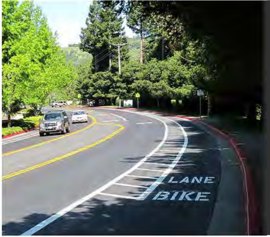
The use of pavement markings delineates space for bicyclists to ride in a comfortable facility.
