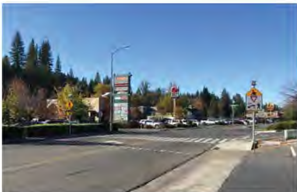
Figure 6-10: Example of an RRFB in Placerville
