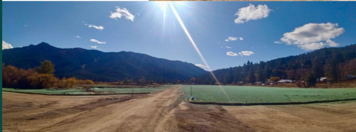
Crescent Mills Phase I Remediation
