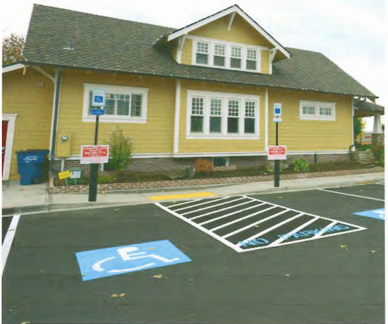
Cones and towing signs line the shared parking lot of the real estate office of Terrie Cox and Chick-fil-A on Southeast Mill Plain Boulevard. (Ariane Kunze/The Columbian)
