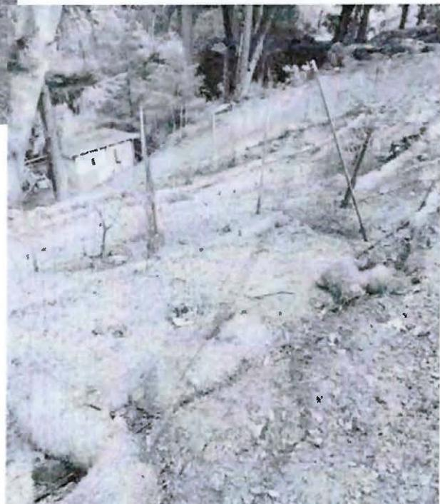
**Figure 4 – Straw waddle placement after EID stripped the upper slope in 2021.**
