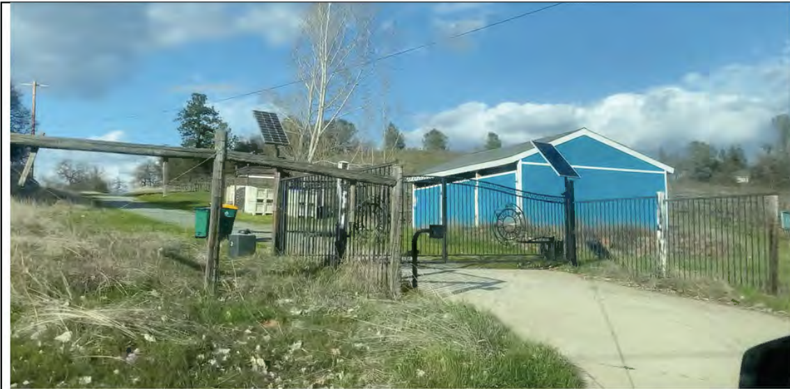
D'Agostini Road at Project Driveway, looking north
