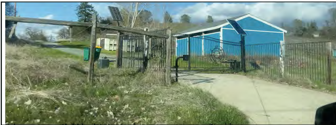
FIGURE 5. PROJECT ENTRANCE DRIVEWAY, DRIVEWAY THROAT DISTANCE
