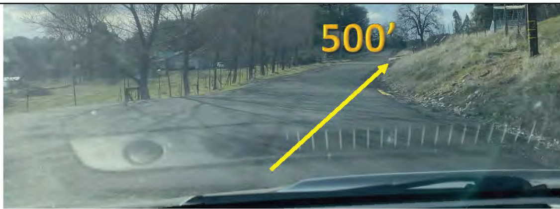
D'Agostini Road Approaching Project Driveway, looking west, has over 500 feet of Sight Distance
