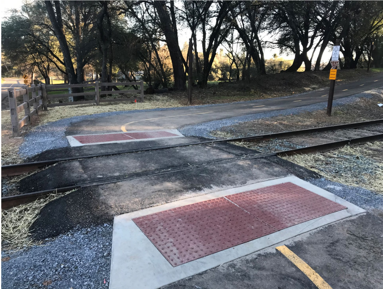
Typical at-grade rail crossing
