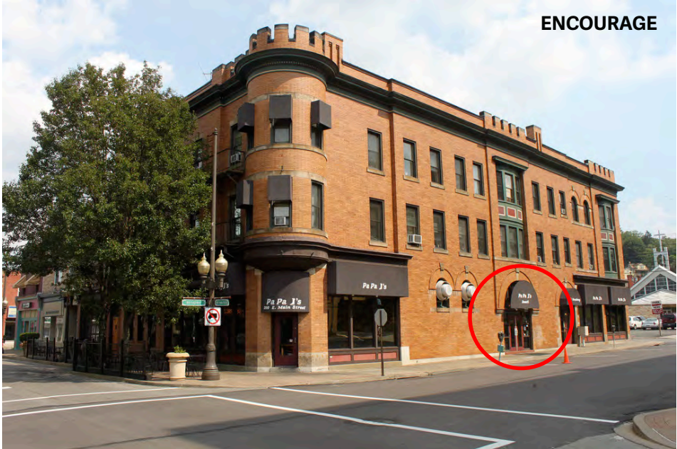
This corner-lot building faces its entrance at the corner and the turret above the entrance signals its location. A side entrance (circled) offers separate access for residential uses.
