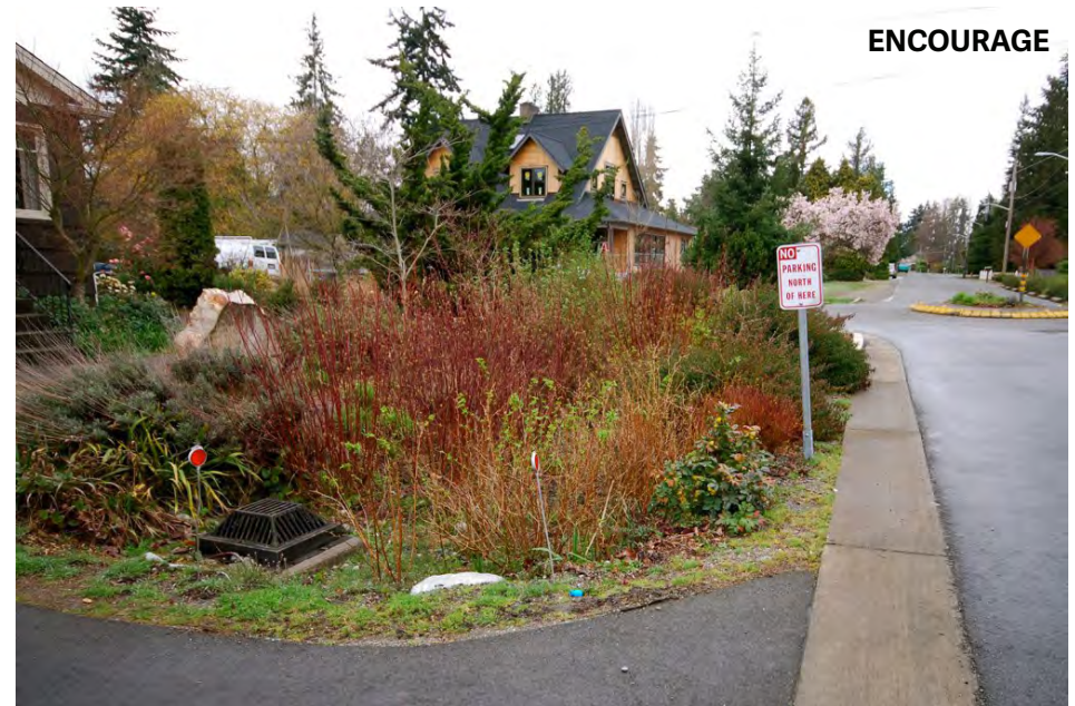
This landscaped area acts as a bioswale. Bioswales remove silt and pollution from surface runoff water.
