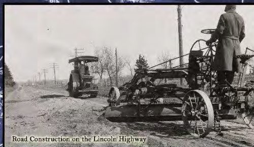
Road Construction on the Lincoln Highway
