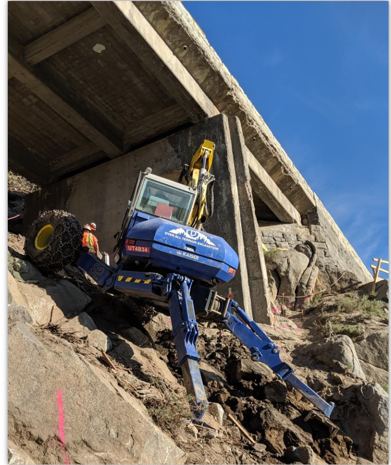
Foundation Excavation
