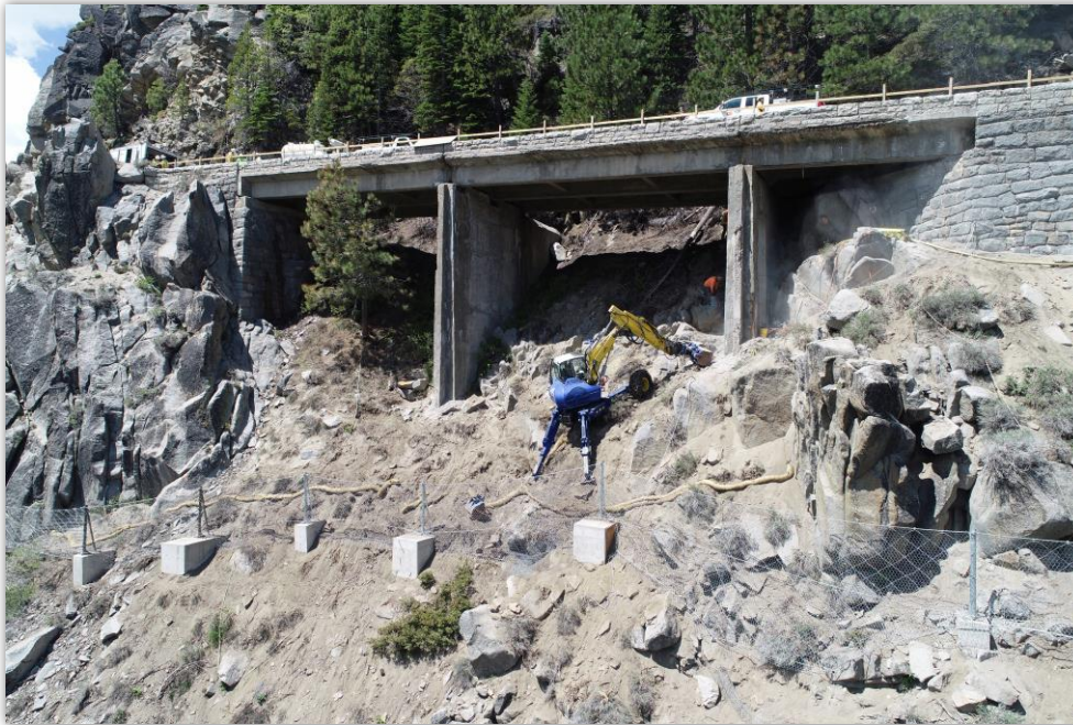
Rockfall protection and excavation
