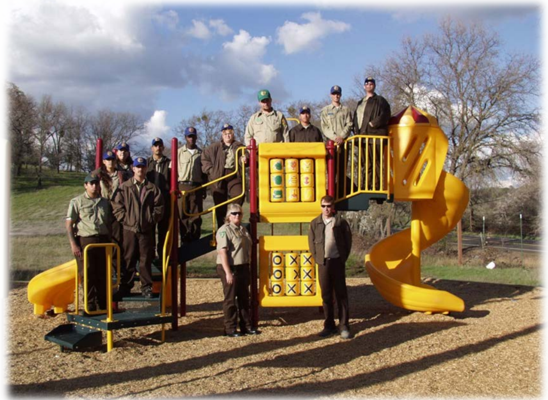
CCC crew at Greenwood constructed the Tot Lot at The Bayley House Park 13-0876 A 14 of 31
