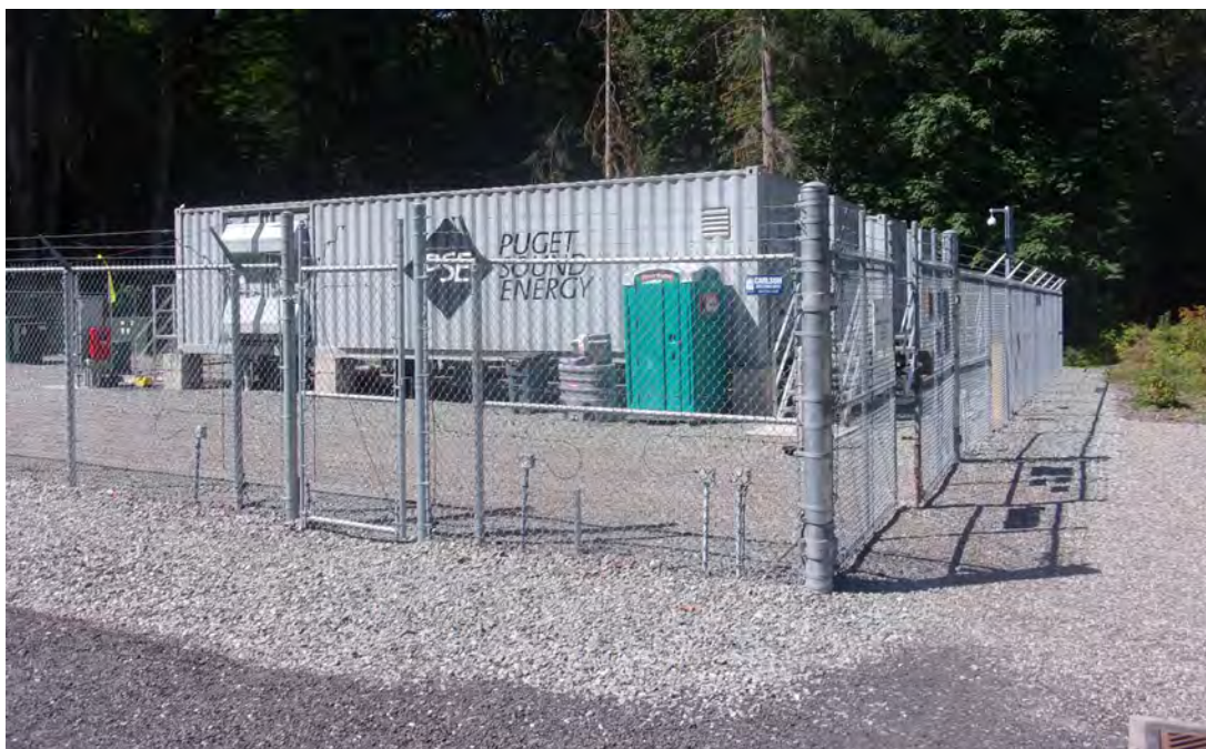
A standalone utility asset battery system at a substation in central Whatcom County, Washington (Credit: Robert Ashworth, Flickr )
