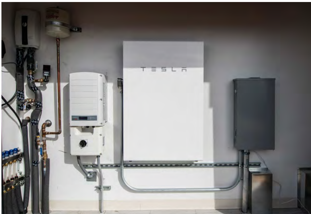
A Tesla Powerwall residential battery system (Photo by Dennis Schroeder, NREL 48520)
