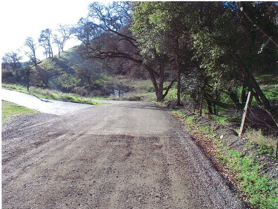
Start of Pavement at MP 3.54 (Project Limit East End)
