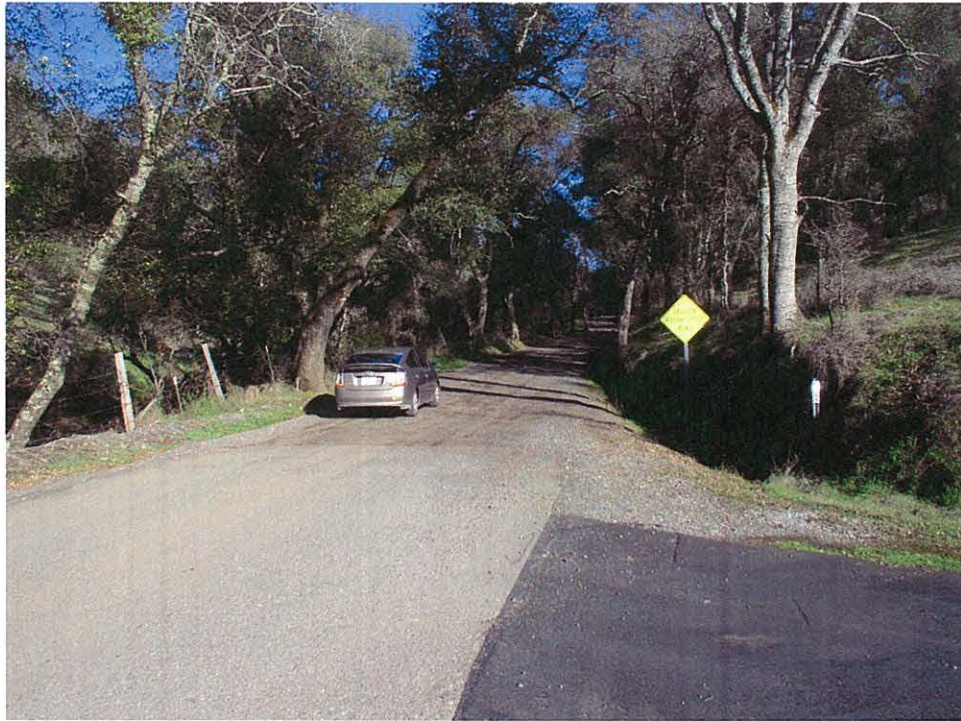
End of unpaved segment at driveway to 6392 Bayne Rd (MP 3.54)
