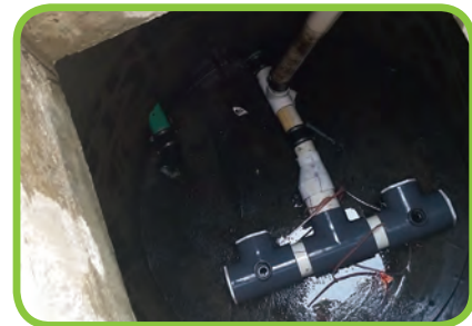
Manifold Tee View of a Cleaned System
