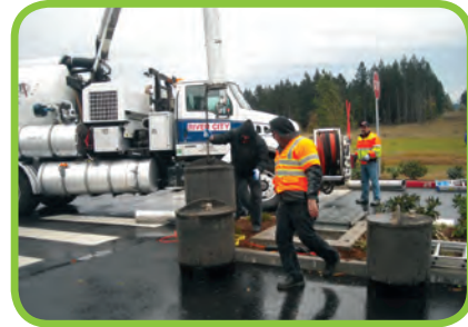
BayFilter System Cleanout
