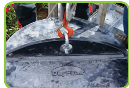
Cartridge Hoist Point
