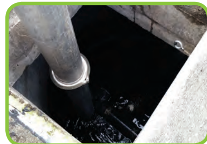
Jet Vactoring Through Access Hatch
