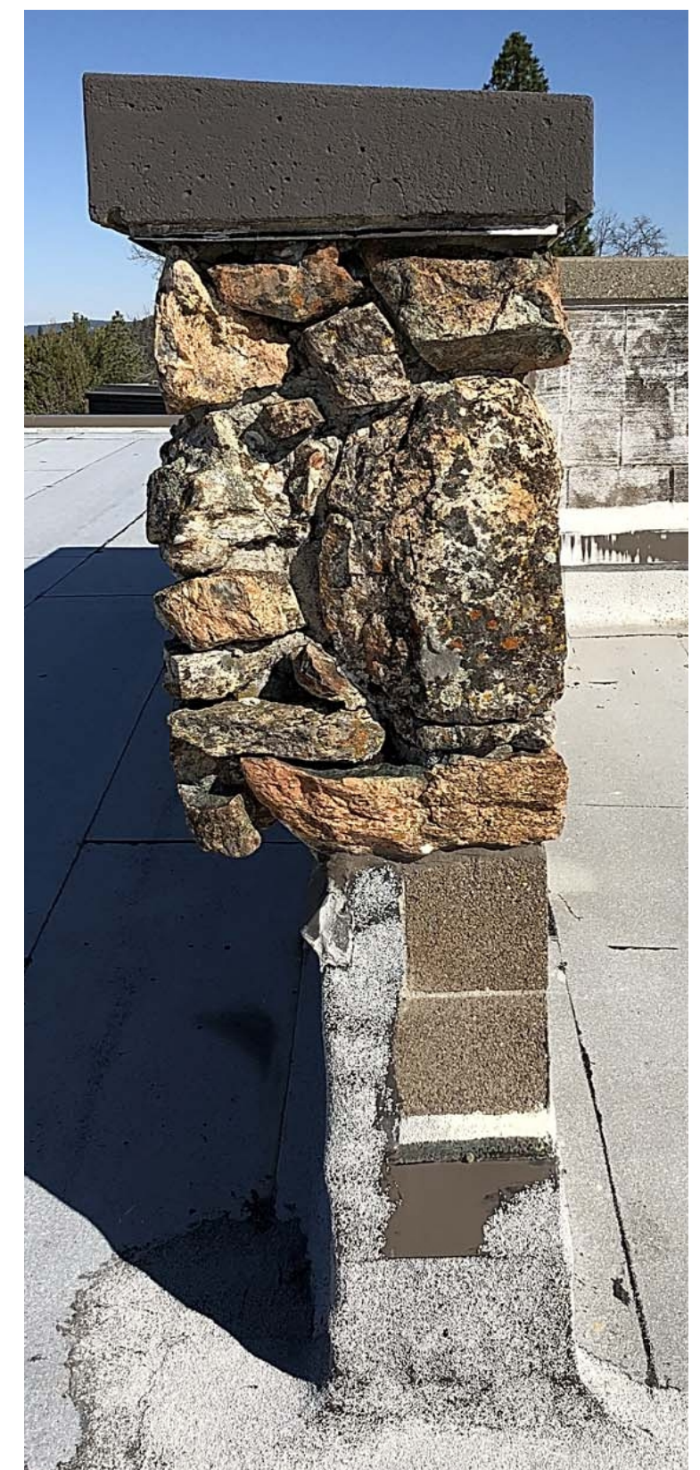
PARAPET SAMPLE PHOTO
