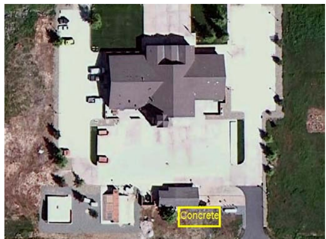
Photo 5. Aerial view of proposed concrete location.
