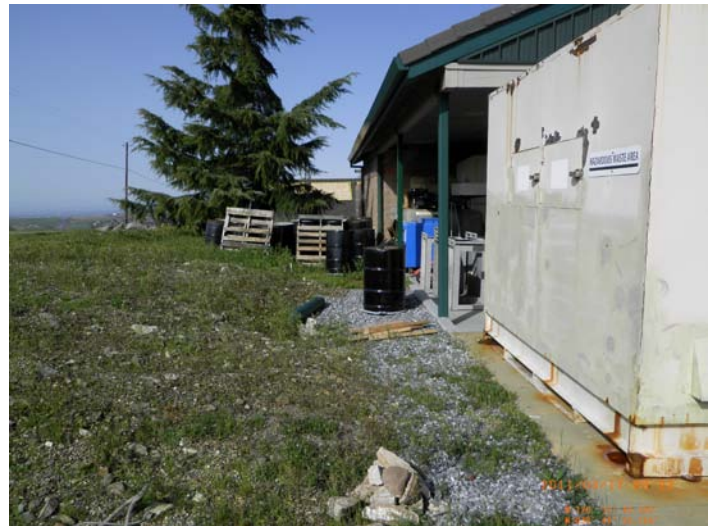
Photo 3. Location for new concrete pad.
