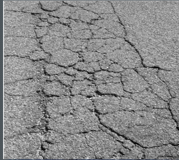
Alligator Cracking
