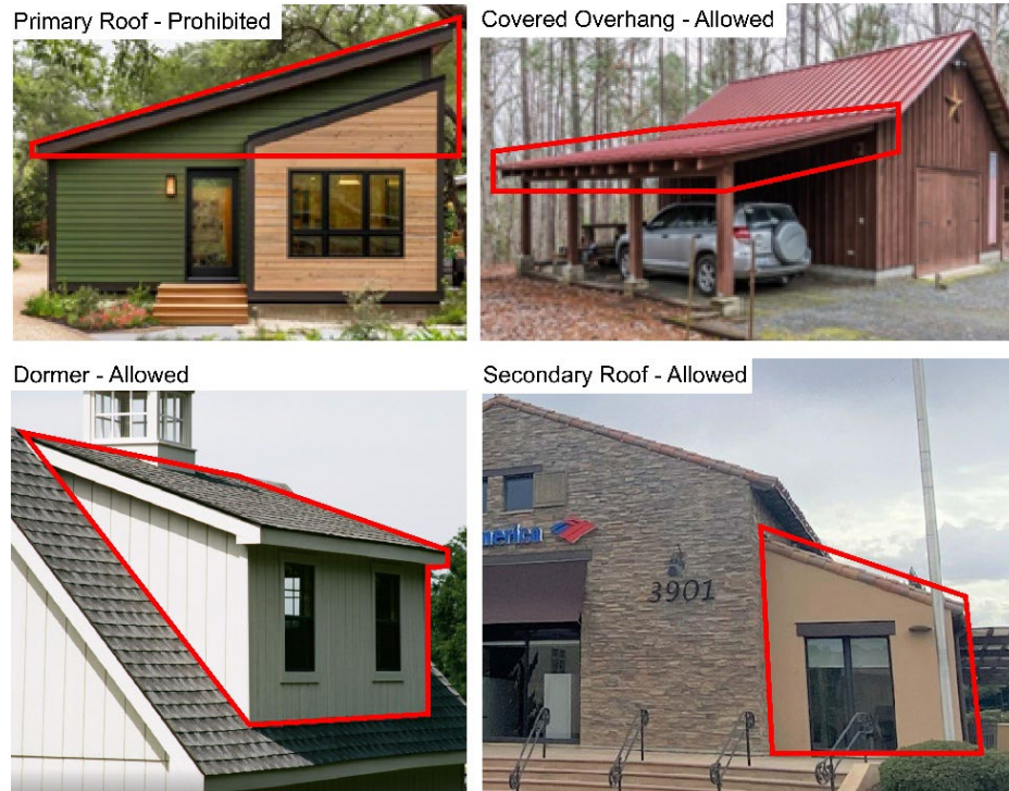
Figure 7 Shed Roof Types
