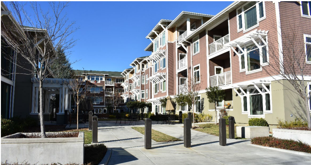
Figure 14 Shared Community Courtyard, Winters, California
