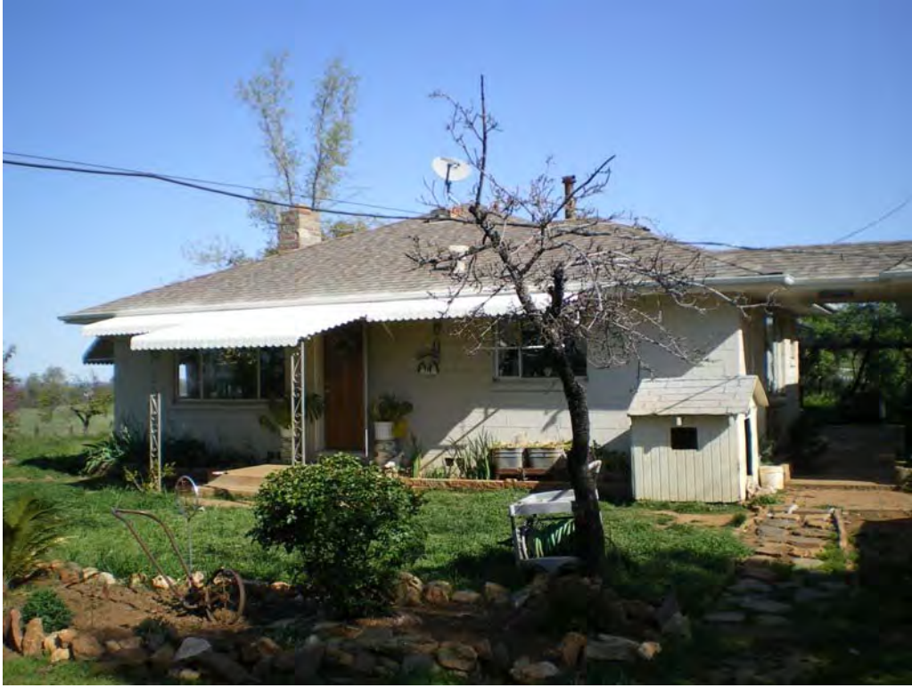
South (front) elevation of residence, view towards north
