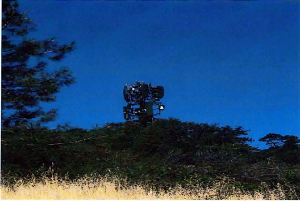
Cell Tower off Arroyo Vista Rd:
