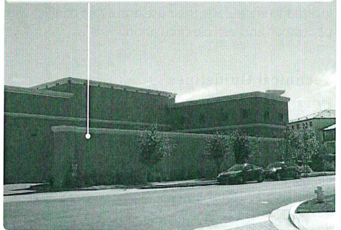
Architecturally integrated screenwall effectively screens loading dock from street.
