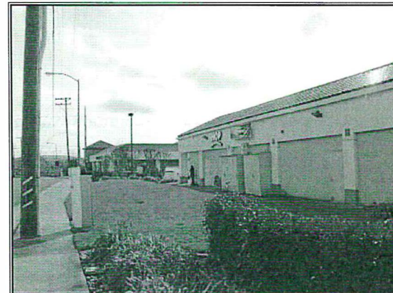
Don't Do This: A commercial project in Folsom, California. The street-facing façade is blank and cold. There is no visibility into the buildings from the street or from the buildings to the street. The structure lacks visual interest and architectural character.
