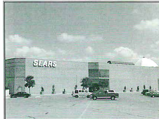
Don't Do This: This commercial building has little facade articulation and appears as one massive building. It ignores the human user.
