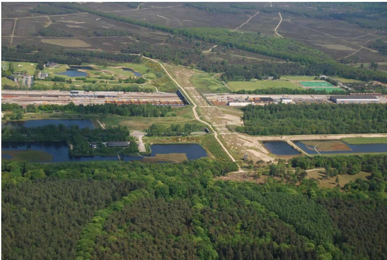
Figure 27. Photo. Most wildlife overpasses or landscape bridges are less than 70-80 m long; however, the one shown above Hilversum, The Netherlands, is 800 m long and spans two roads and a railroad. (Credit: Goois Natuurreservaat, The Netherlands/Photo: W. Metz).
