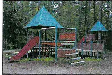
Traditional structures painted to blend with the surroundings are recommended.
