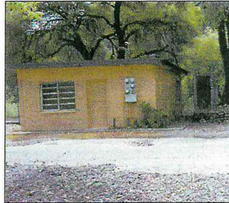
Existing restroom facility.
