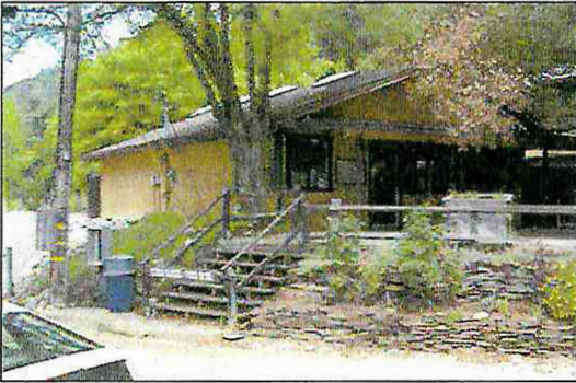
Existing store facility.
