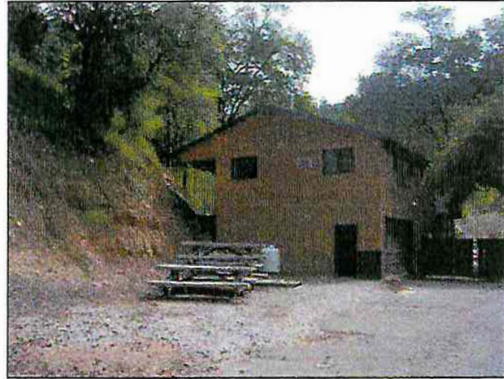
A rooftop deck over storage would provide needed access to the upper level of the house.
