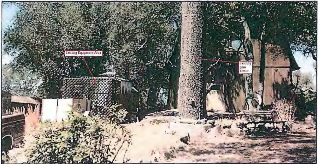
Photo of Existing SBA Ground Equipment
