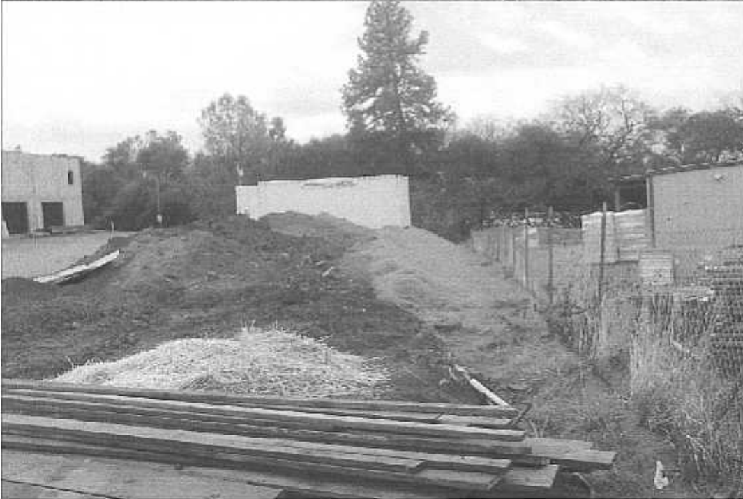
Comment: Boundary to north of Building B, feed store (commercial) to the right
