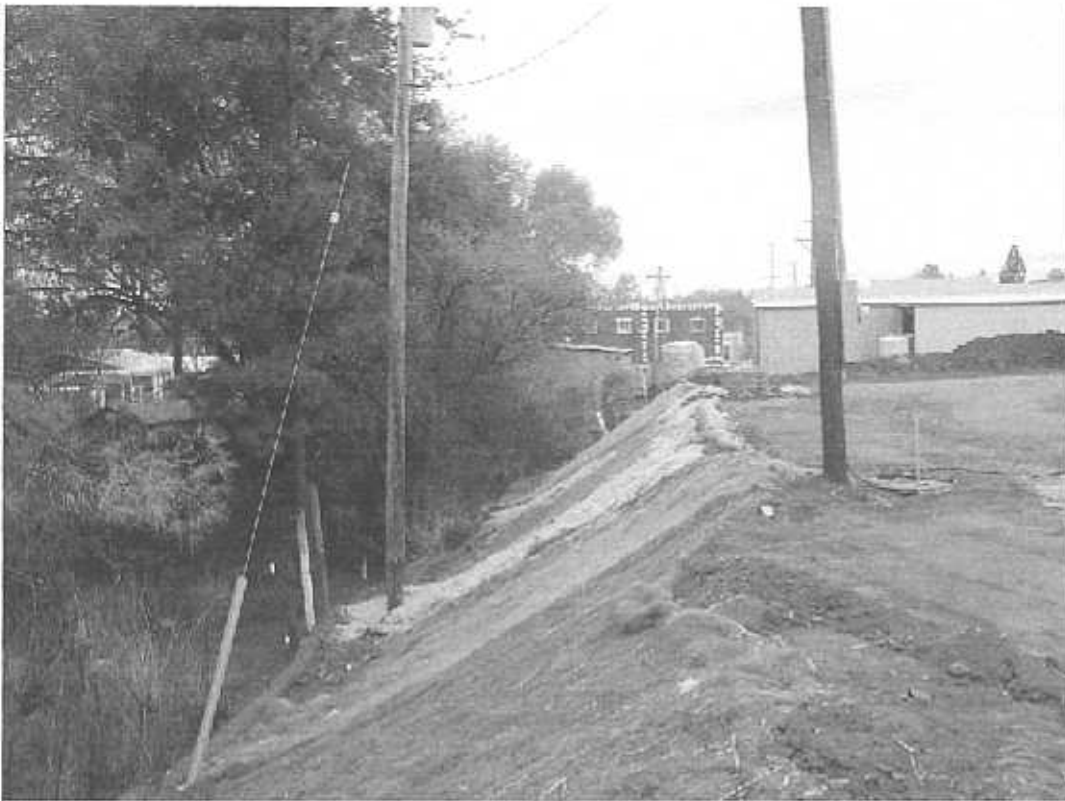
Comment: West boundary beside Building B next to residential zone
