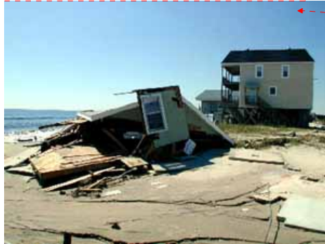
Hurricane Floyd brought a devastating 15 feet of storm surge that damaged or destroyed hundreds of houses along the ocean front of Long Beach on Oak Island, North Carolina in September 1999. A prime example of successful hazard mitigation, the elevated home (right) survived while the older, ground-level block foundation of the home on the left was crushed.
