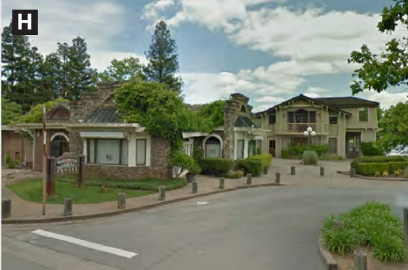
H This horizontal mixed use development features retail, offices, and residences spread across one parcel.
