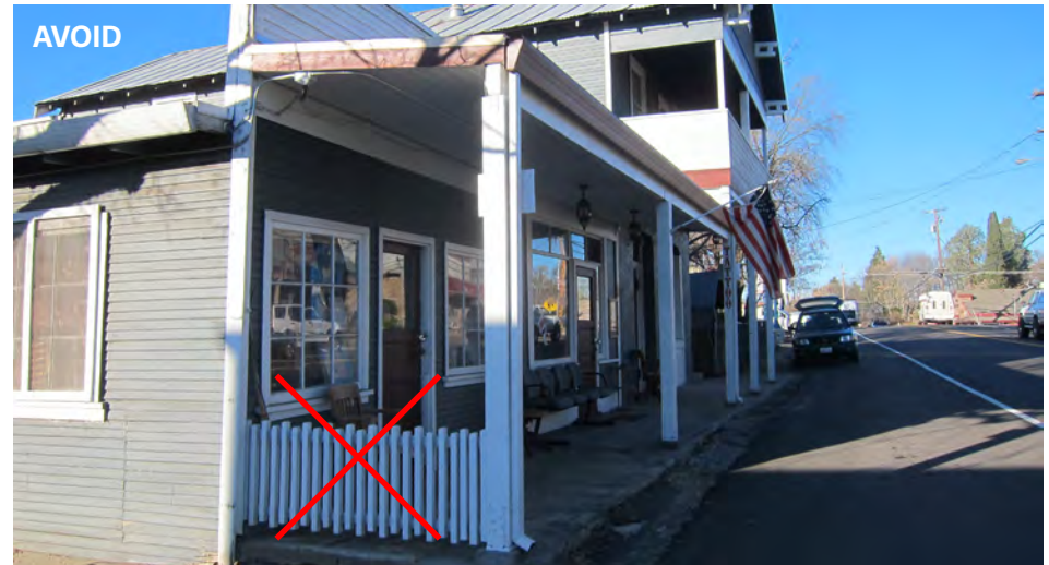
Arcades create protected pedestrian zones and shape the character of El Dorado County. Restricting access poses a safety risk.
