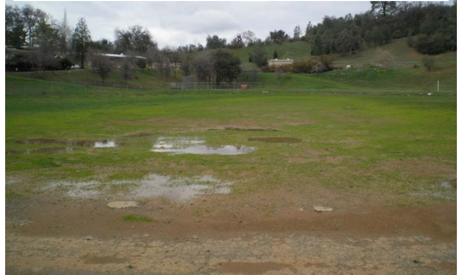
Drainage at large field
