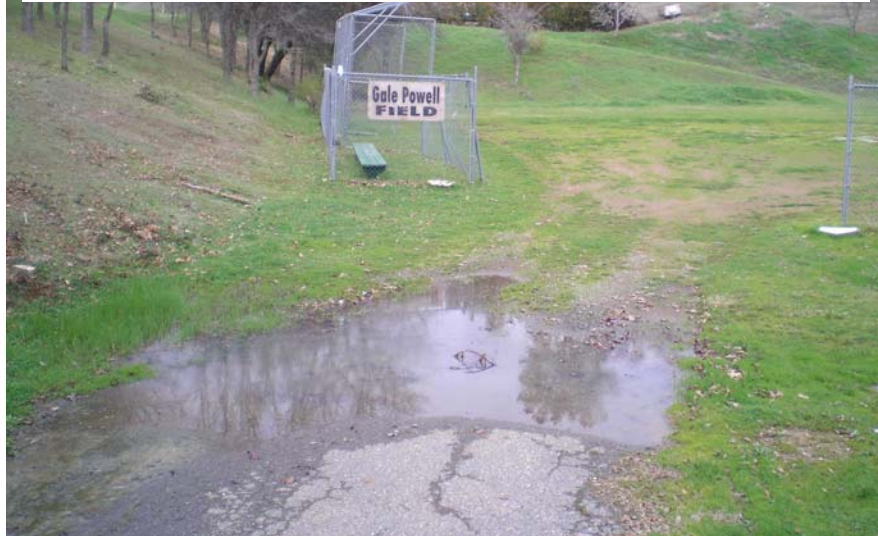
Drainage at small field
