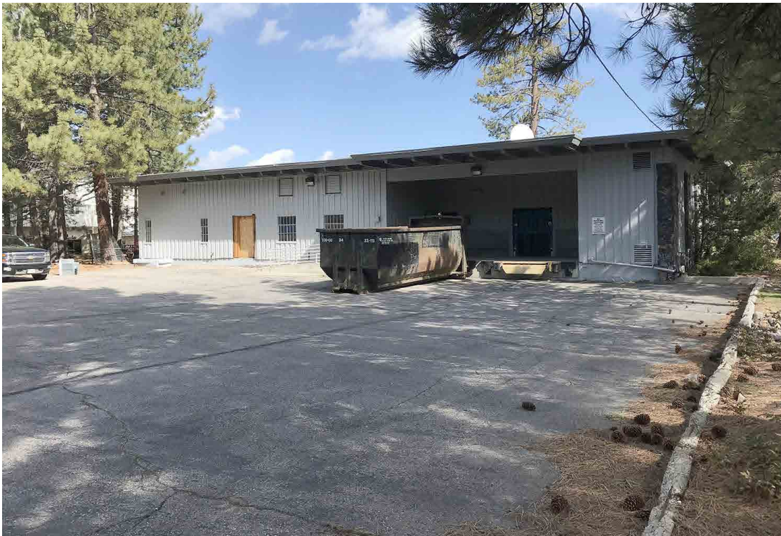
Photo No. 2 Rear parking lot and loading dock
