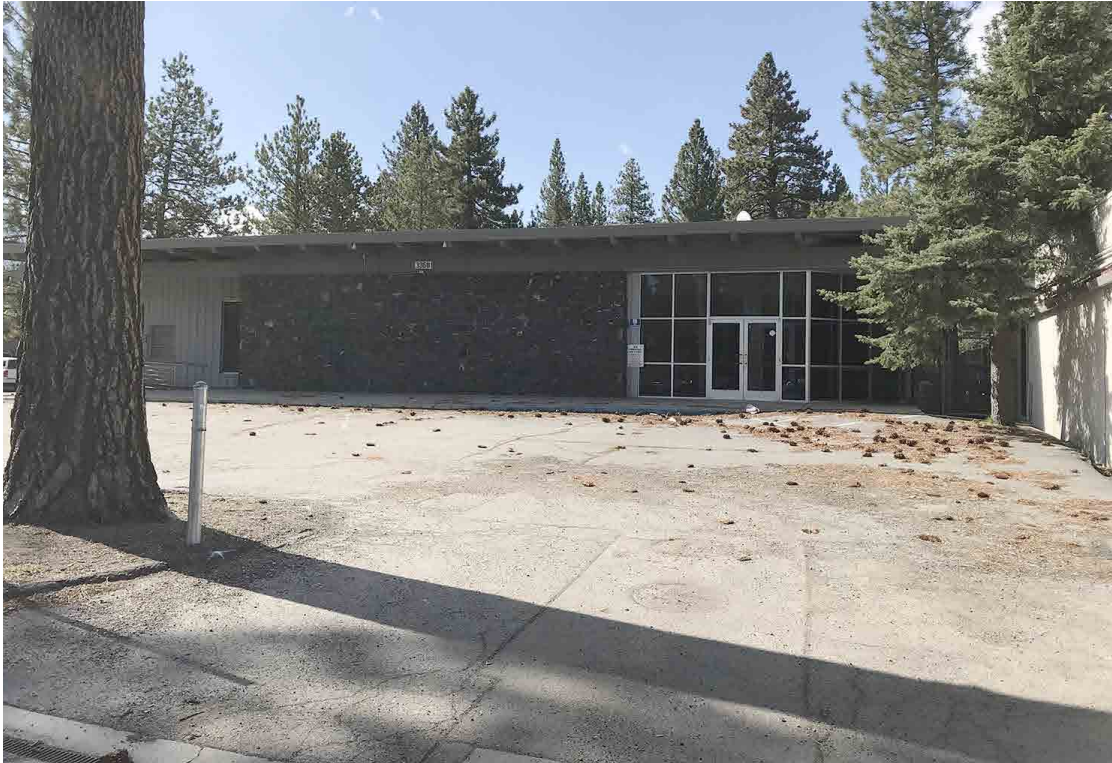
Photo No. 1 Front parking lot and building entrance
