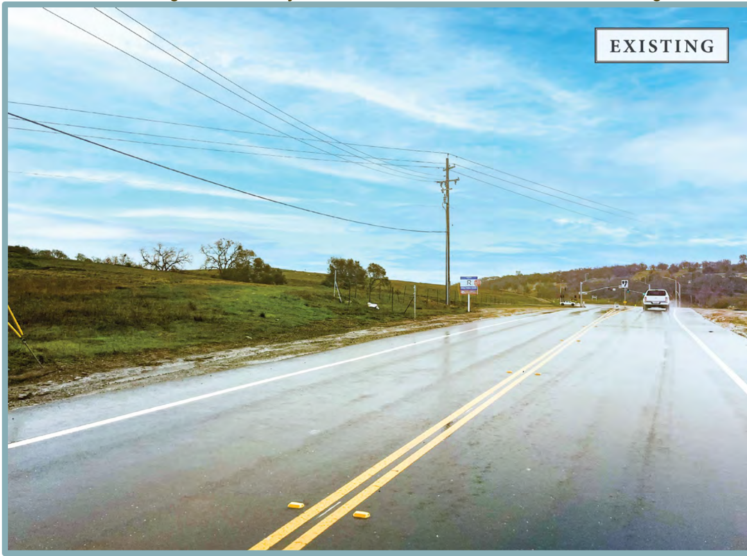
Figure 4.1-7 View 4: Existing View of Project Site from the Bass Lake Road Looking South
