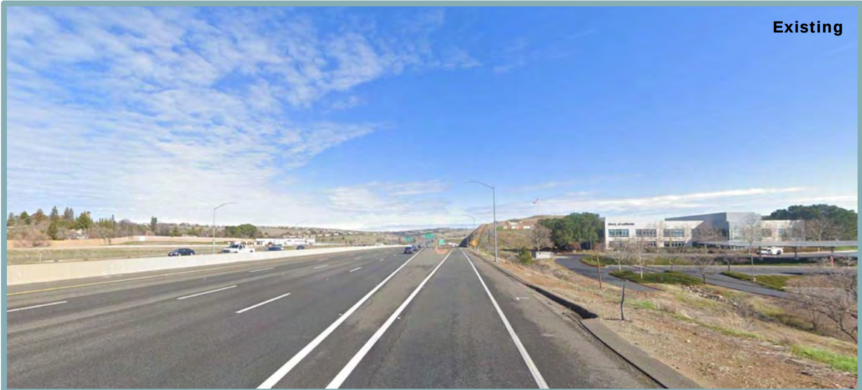
Figure 4.1-12 View B: Existing View from Eastbound US 50 and El Dorado Hills Boulevard Off-Ramp Looking East
