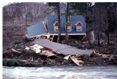
Photo 2: Cabins damaged and destroyed by the massive Mill Creek landslide that occurred on January 24, 1997. USGS Photo by Mark Reid, USGS/Menlo Park, 1997
