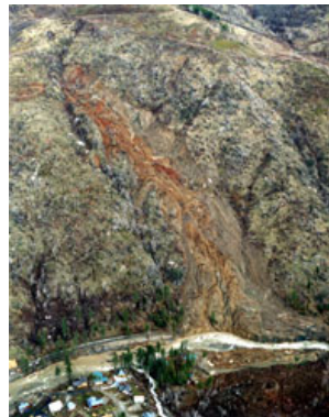
Photo 1: Aerial view of the Mill Creek landslide blocking Highway 50. Caltrans Photo courtesy of Lynn Harrison, Caltrans
