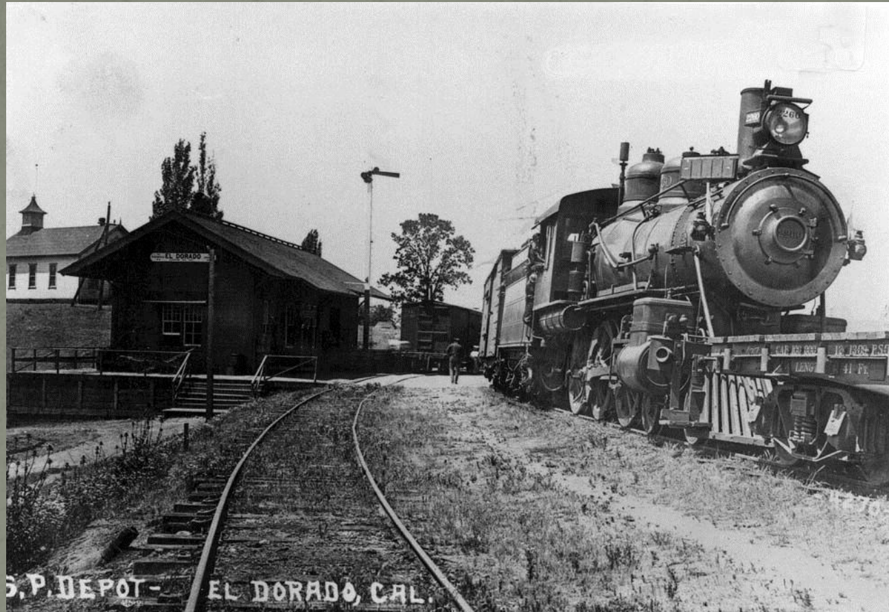
Historical photograph of the 1888 El Dorado Station with the El Dorado School, now the Community Hall, on the left.
