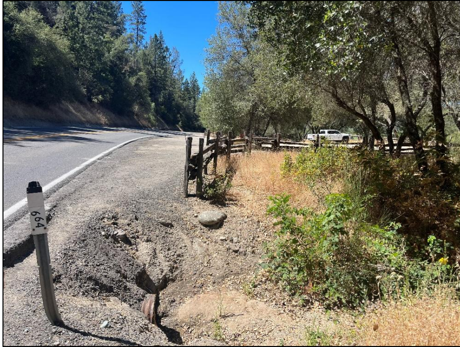
Photo 3. Representative photo of a culvert along Lotus Road that is to be reinforced with RSP to prevent further soil erosion from large rain events. Taken facing south (8/13/2024).
