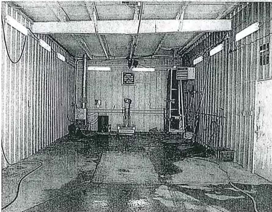
Floor drains in service bays might lead to a Class V (Five) Motor Vehicle Waste Disposal Well.
