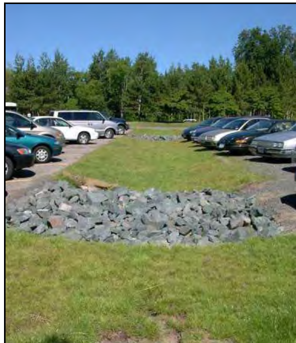
Grassy swale used to filter parking lot runoff
