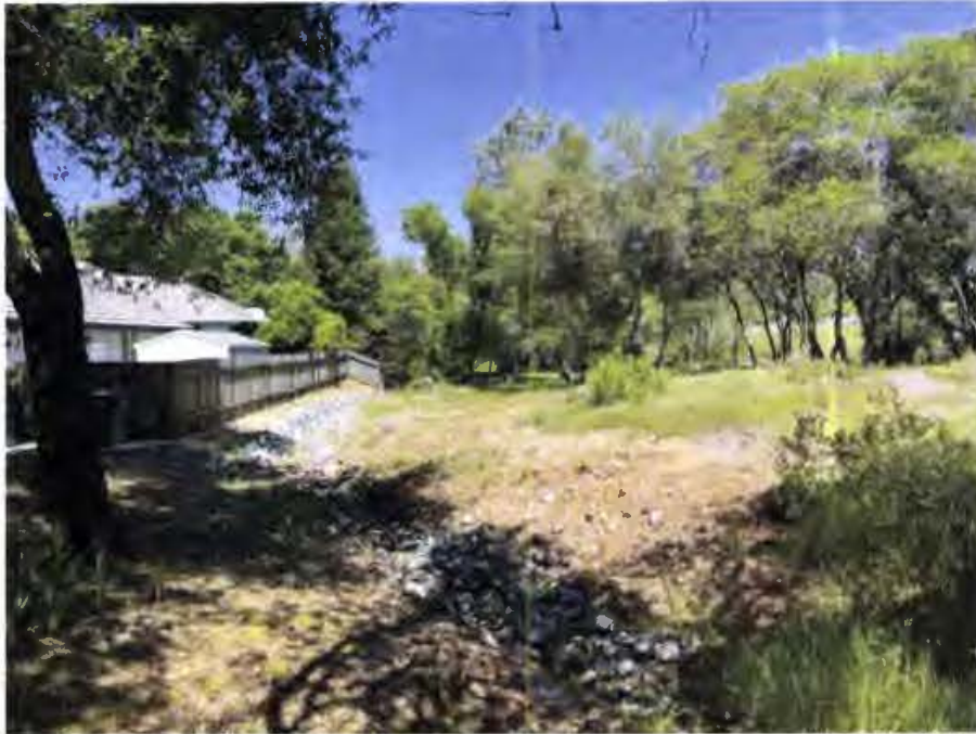
Photo 5. Armored stormwater drainage along western edge of parcel. (5/10/23)
