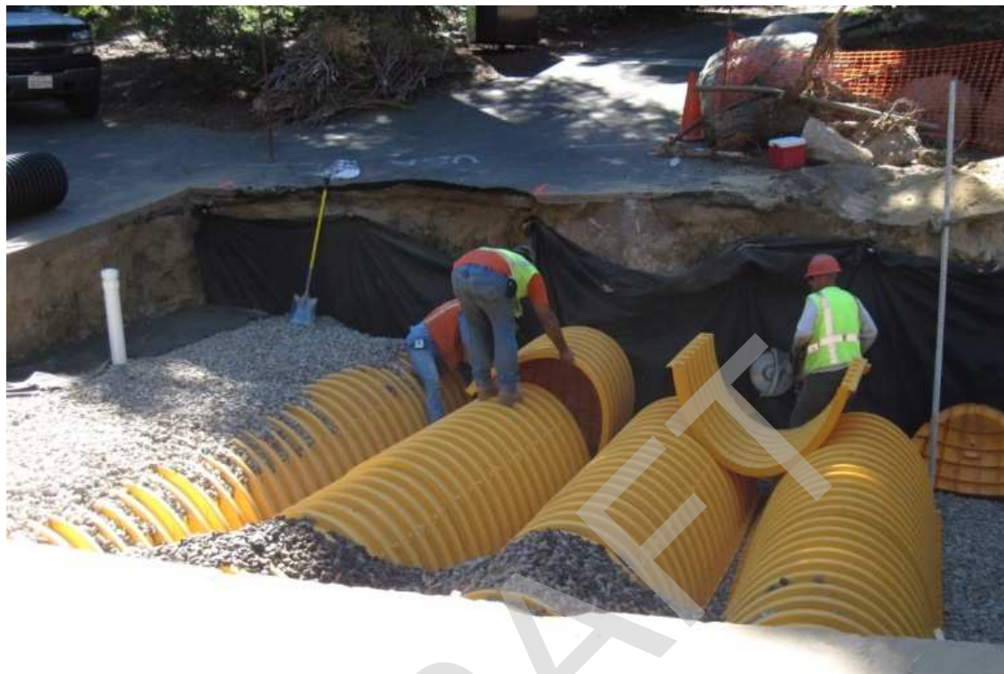
Figure 10: Rubicon Stormtech chambers during installation, 2010 (photo courtesy of El Dorado County).
