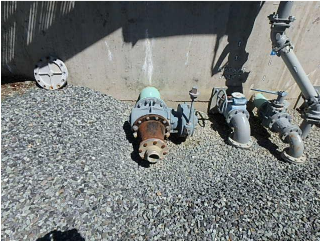
On-site Recycled Water Hook Up
