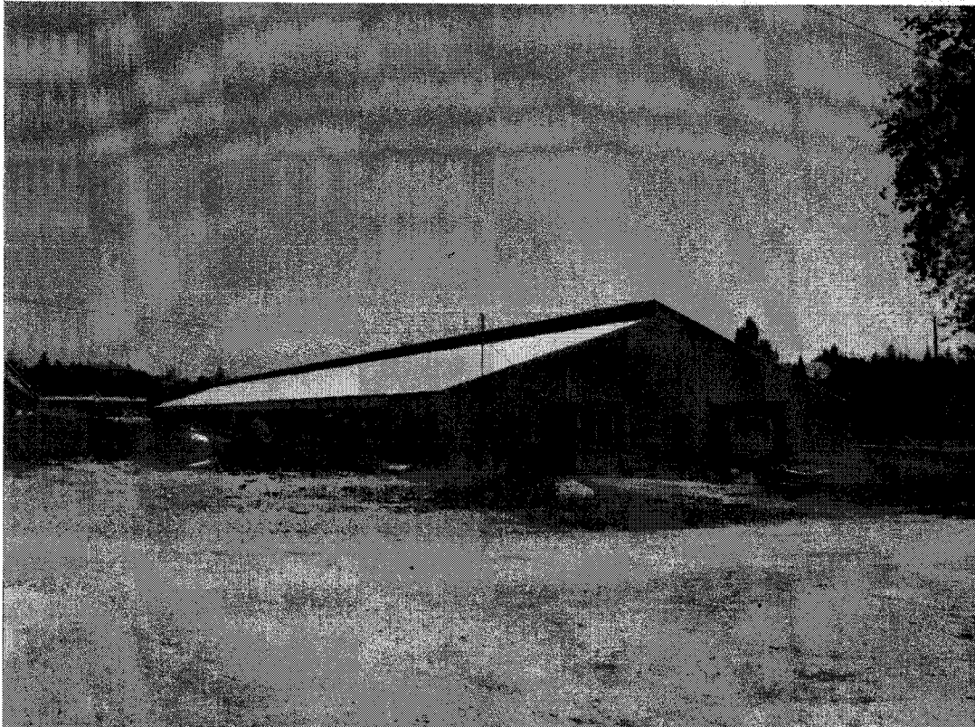
Comment: Building 1 looking from the northwest
