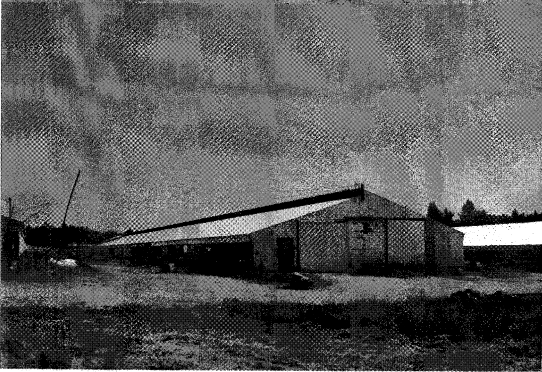
Comment: Building 2 looking from the northwest
