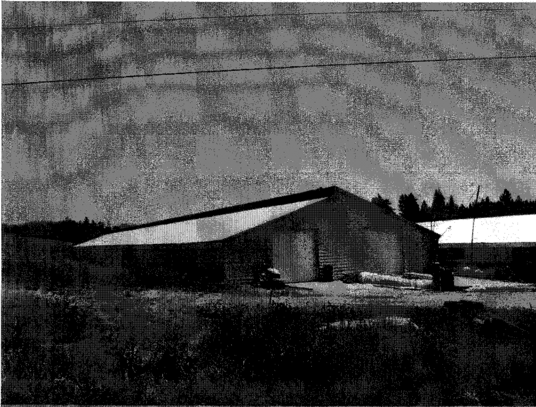
Comment: Building 3 looking from the northwest.
