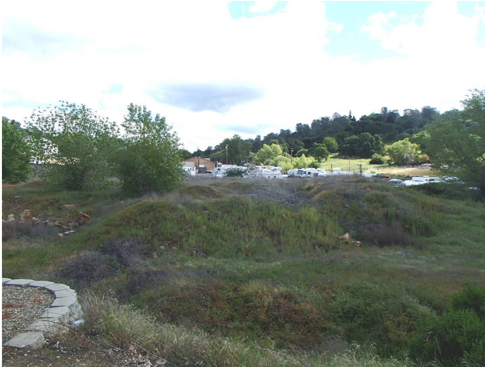
Photo 3.2-1. View east from the edge of Sophia Parkway. Spoils piles left over from the construction of Sophia Parkway and widening of Green Valley Road in 2002 are visible. (Source: Sycamore 2015)
