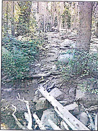
Before: (looking at trail, north of Meeks Creek) erosion damaged, steep grade caused further erosion.
