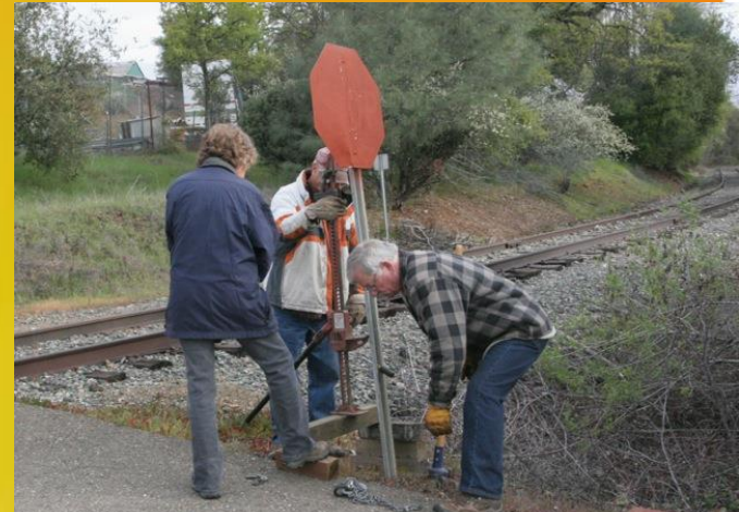
Installing stop sign at a private road crossing
