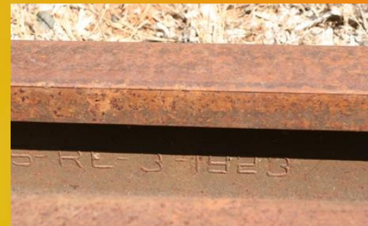
1923 stamped on rail near Missouri Flat Rd
