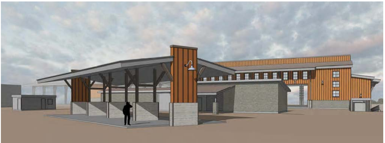
Waste Connections Recycle Canopy
