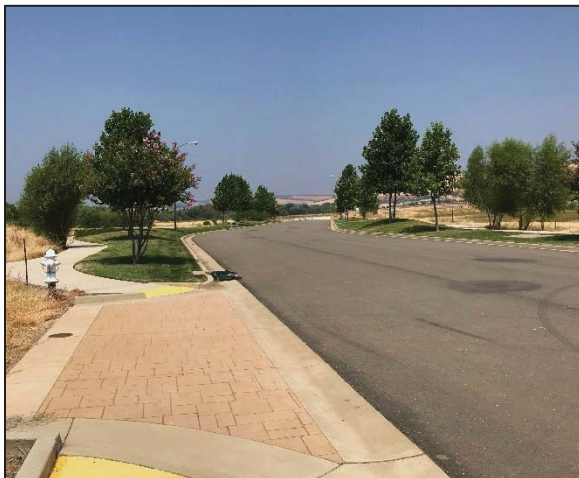
Constructed portion Carson Crossing Drive Extension
