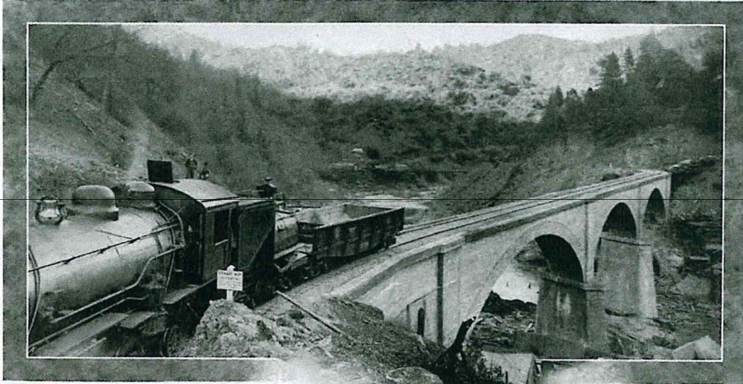
This bridge stands 75 feet above the river, and the skew or angle of the bridge across the river is here plainly seen. Note the heavy Mallet compound engine, indicating unusual demand upon the structure
