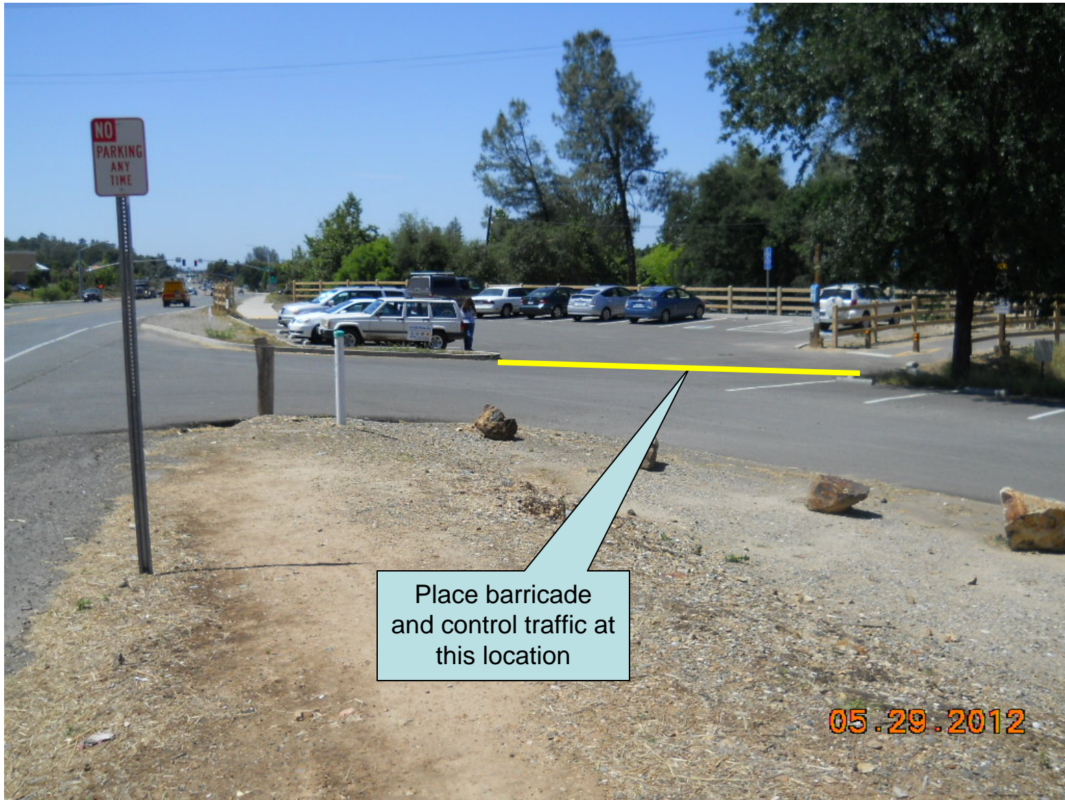
View from Right Side of Parking Lot: Place barricade at curb return to parking stall on right.
