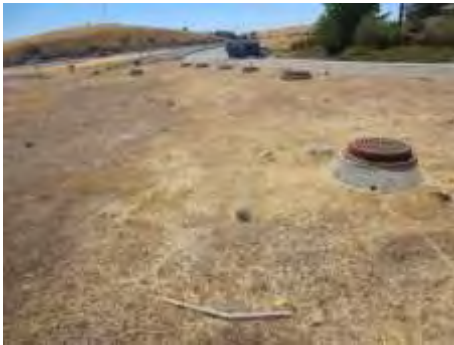
UTILITIES ON SUBJECT PROPERTY LOOKING SOUTHWEST
