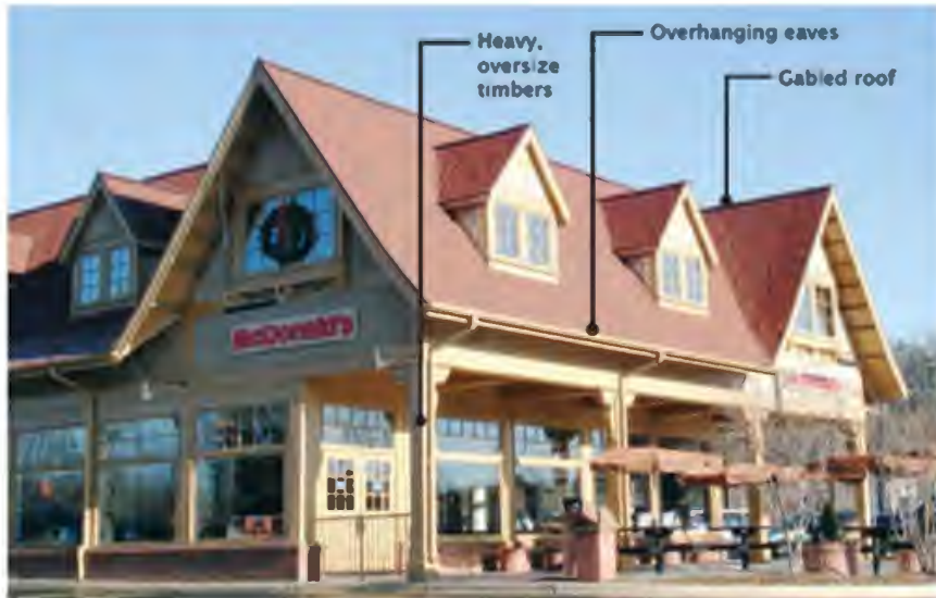
Figure 2. Typical Design Features of the Mountain/Lodge Style
