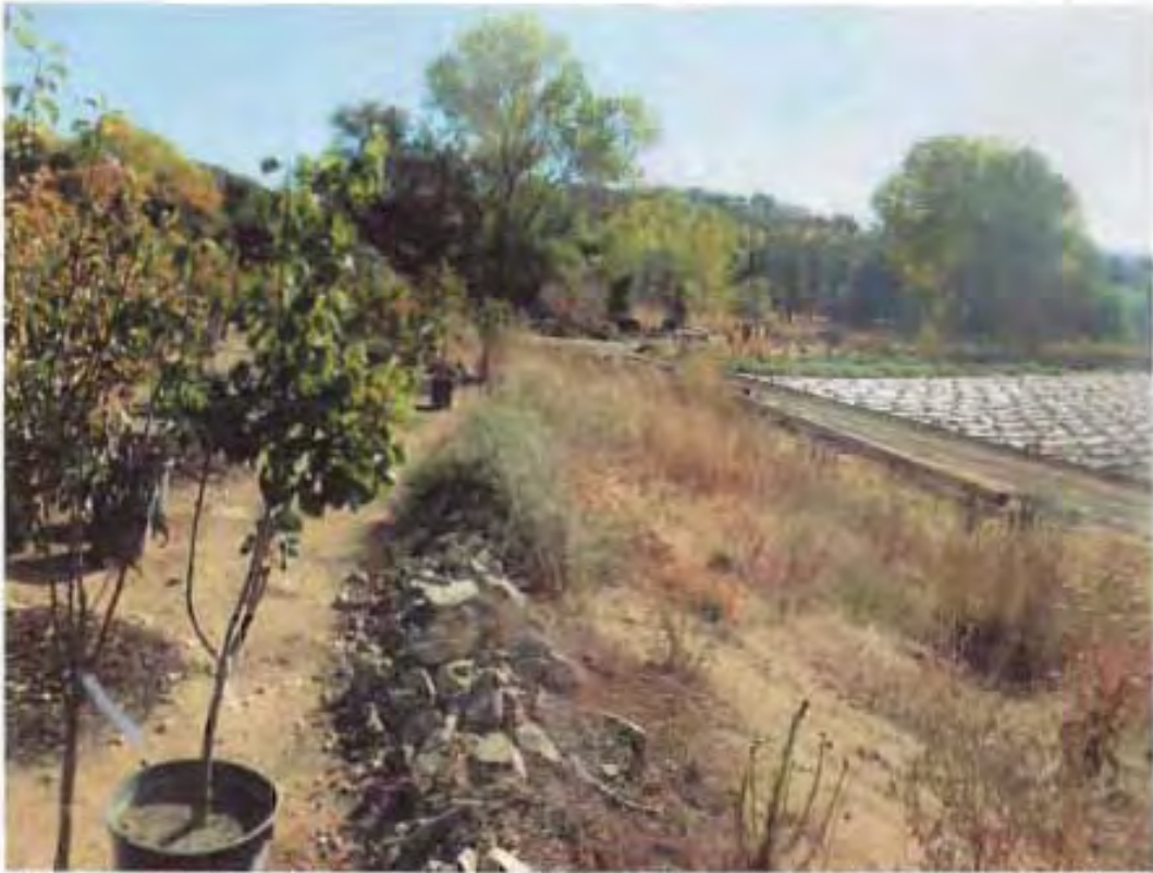
Photo 1. View looking east from the edge of the Nursery. The wetland swale is at the bottom of the slope on the right. The rock berm is in the center foreground.
