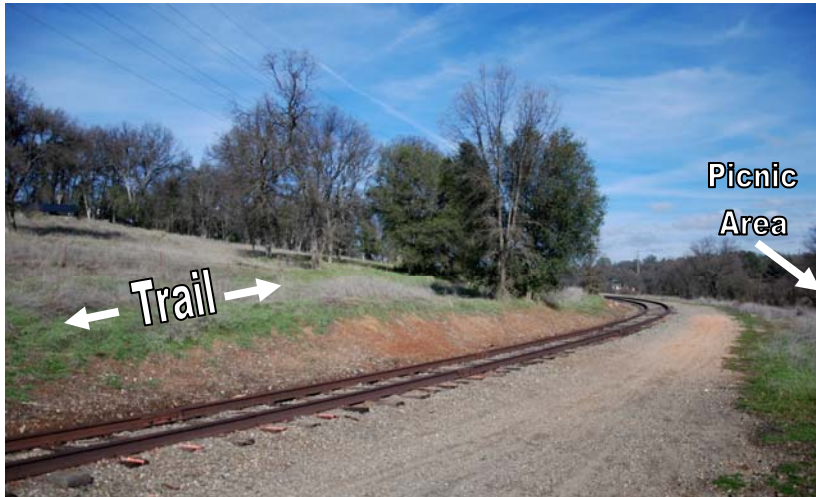
Park Project Site facing northeast
